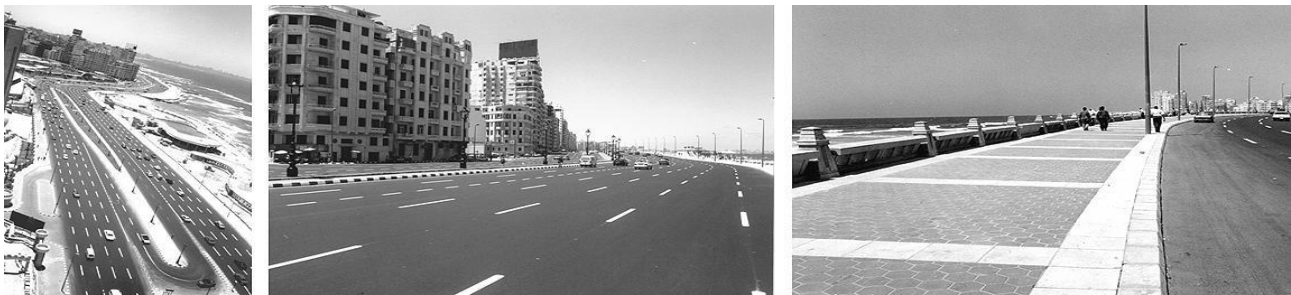
(a) The Cornich as an edge. (b) Widening the Cornich to facilitate traffic. (c) Lack of human features.
